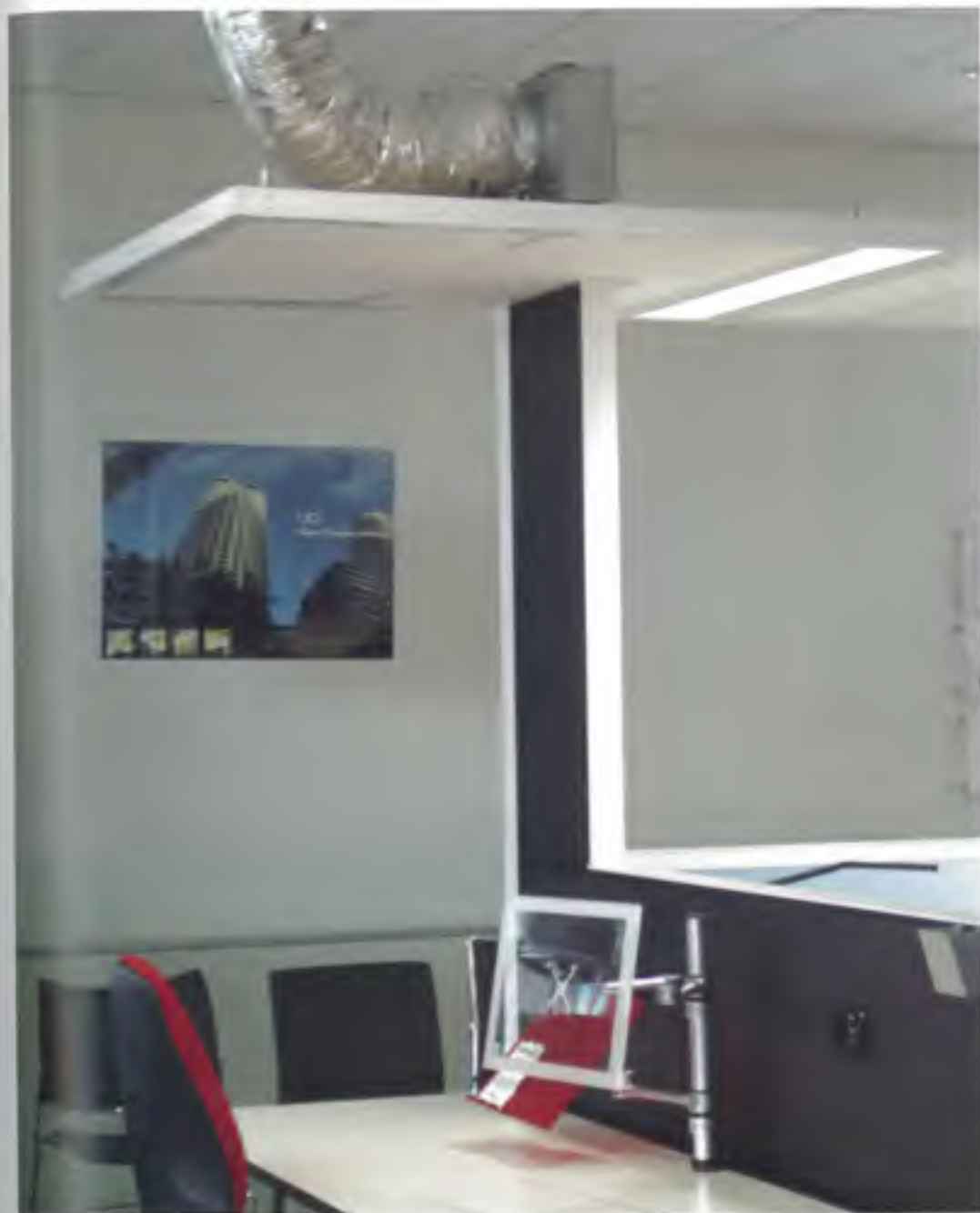
left: Conventional air-conditioning connects to the Task Air workstation via a conventional cushion head.
